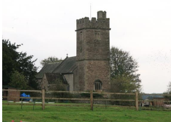
Fig.19 The Church of St Stephen and St Tathan: a mix of ashlar and coursed rubble stone with natural slate roof
