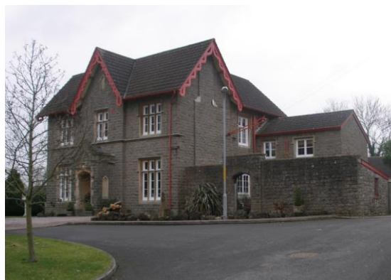
Fig.53 The former Vicarage, outside the walls, is a severe but well designed neo-Tudor building of 1845-6. It appears that its chimneys were removed at a later date.
