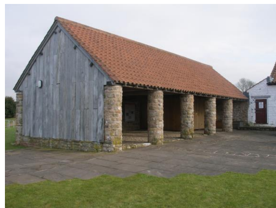
Fig.55 The recently, sensitively converted buildings providing a visitor facility and information point
