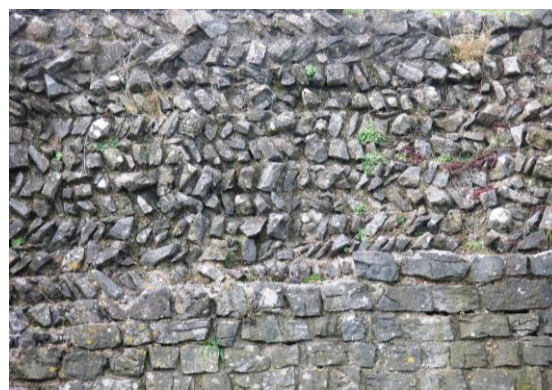
Fig.47 A detail of the Roman wall showing the herringbone stonework of the core structure and the facing stonework
