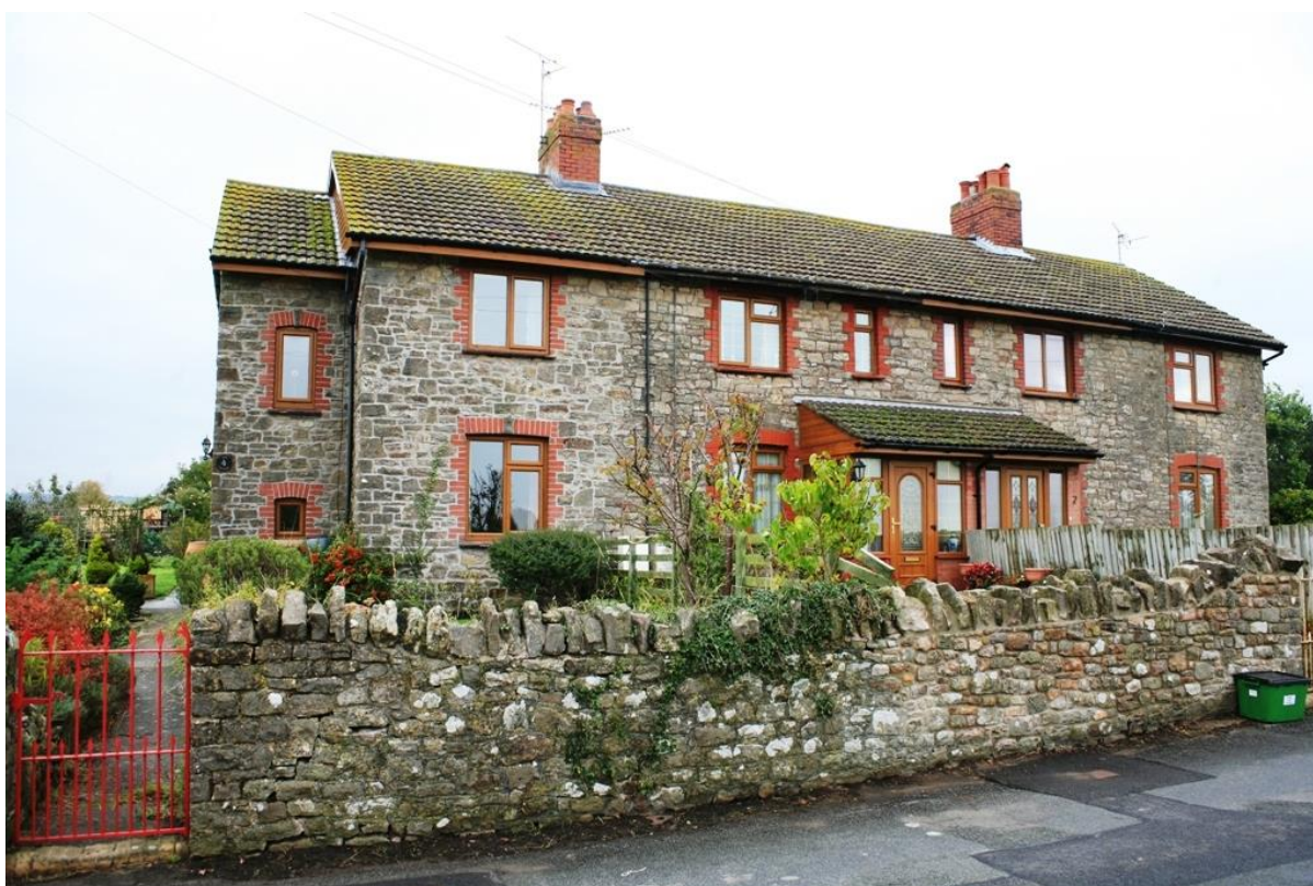
Fig.37 Modern windows and roof covering to New Cottage
