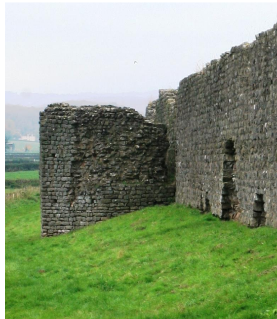
Fig.12 Bastion on the south wall projecting over the town ditch
