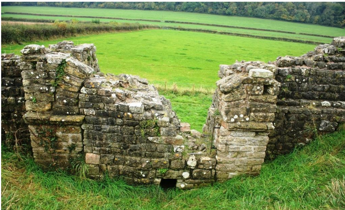
Fig.25 Ruinous South Gate with later Roman stone infill
