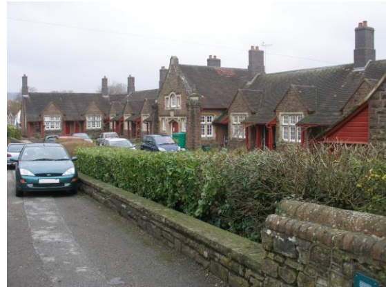
Fig.54 The Burton Almshouses (1913) are a good example of the rather eclectic mix of Arts and Crafts and Arts Nouveau styles prevalent at the time
