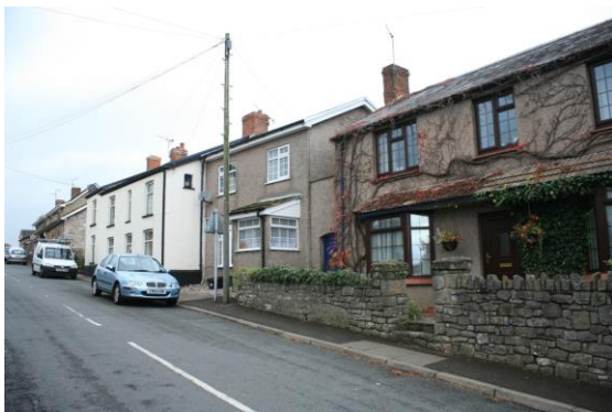
Fig.28 Strongly defined townscape in the village core section of the Conservation Area
