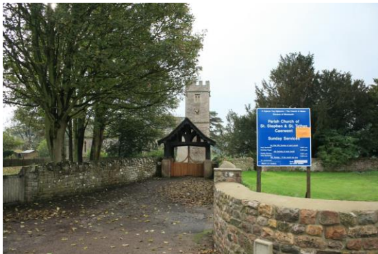
Fig.15 Stone walls are a strong feature of this part of the Conservation Area and in this case form a group with the lych gate of the church
