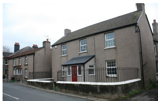
Fig.32 Some survival of iron railings to front boundaries
