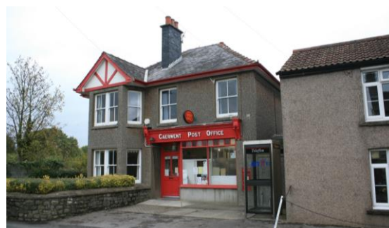
Fig.29 Caerwent Post Office - a good early 20 th century timber shopfront
