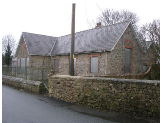
Fig.52 The former Village School: this robustly detailed late Victorian building is now used as a nursery
