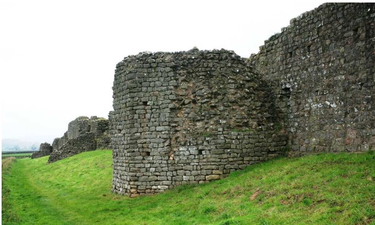
Fig.21 Sandstone block facings to the southern sections of the Town Wall within this part of the Conservation Area.
