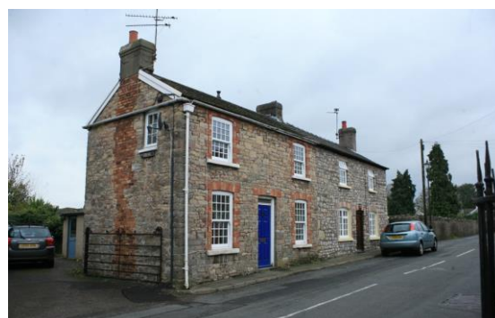
Fig.31 Roughly coursed stone with brick dressings and wrought iron gate to Weston House
